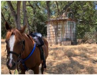
Joseph D. Grant County Park Brush Trail Water Tank
