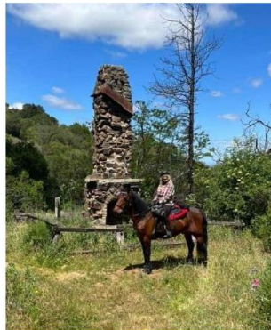
Almaden Quicksilver County Park English Camp Chimney & Vault
